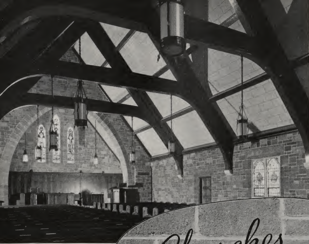
Left —Concrete masonry units, laid up in a combination of random and coursed ashlar, form the walls of the First Presbyterian Church, Plymouth, Michigan. Special shapes were required for arches, jamb returns and window lancets. Thomas Moss, architect.
